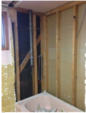
Exterior and interior walls not insulated
